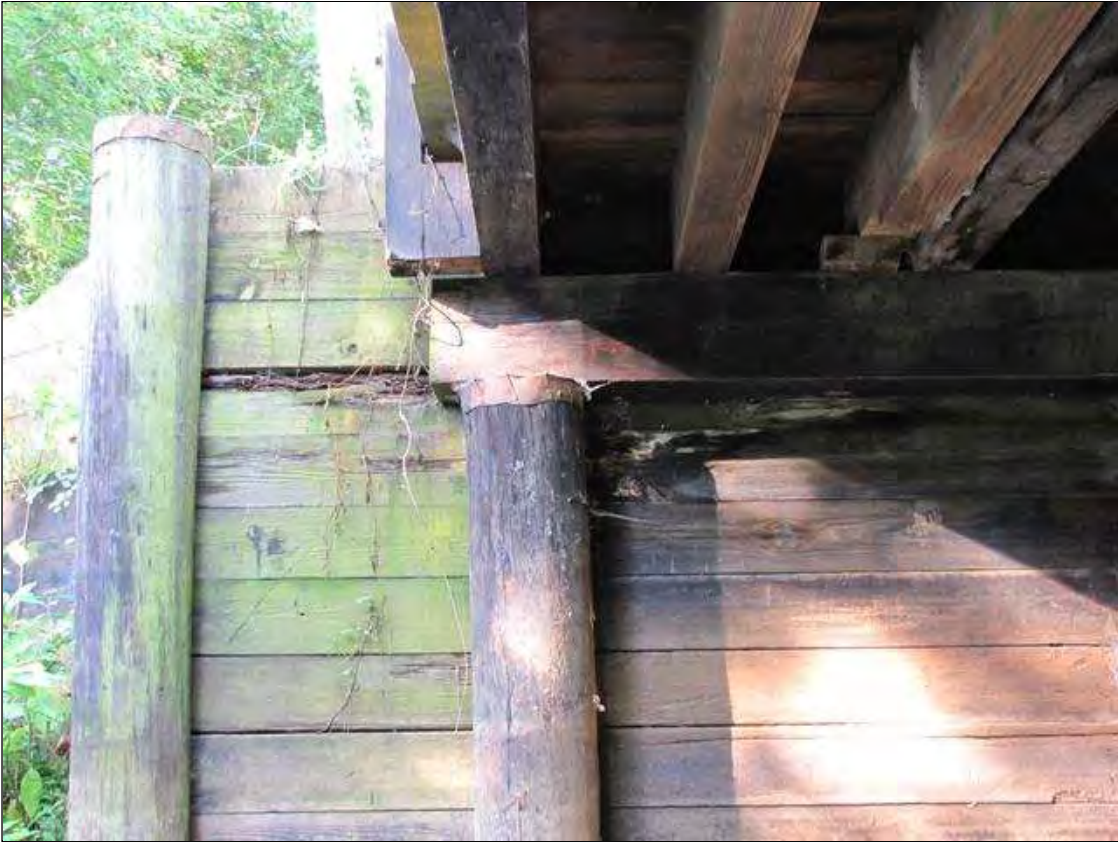
End Bent 1 Abutment/Backwall : 5 FT X 1 FT AREA OF DECAY IN RIGHT END.
