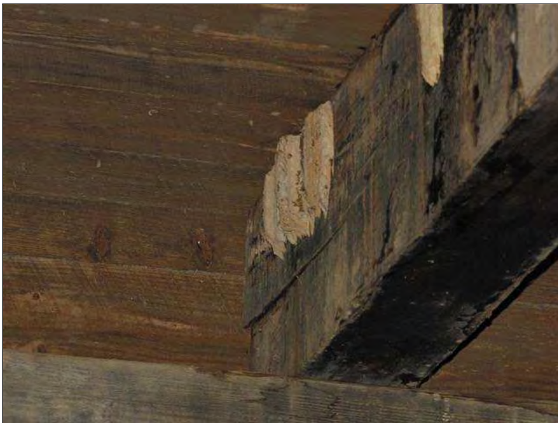
Span 1 Beam 8: 14 IN OF END DECAY WITH CRUSHING UP TO 1 1/2" AT END BENT 1 CAP.
