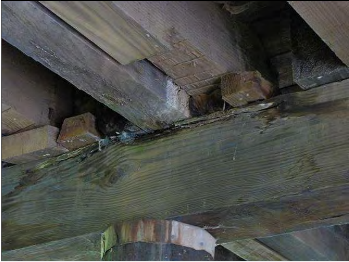
Bent 1 Cap : 3 FT OF CRUSHING AT TOP OF CAP AT BEAMS 4 AND 5 ON SPAN 1 SIDE.
