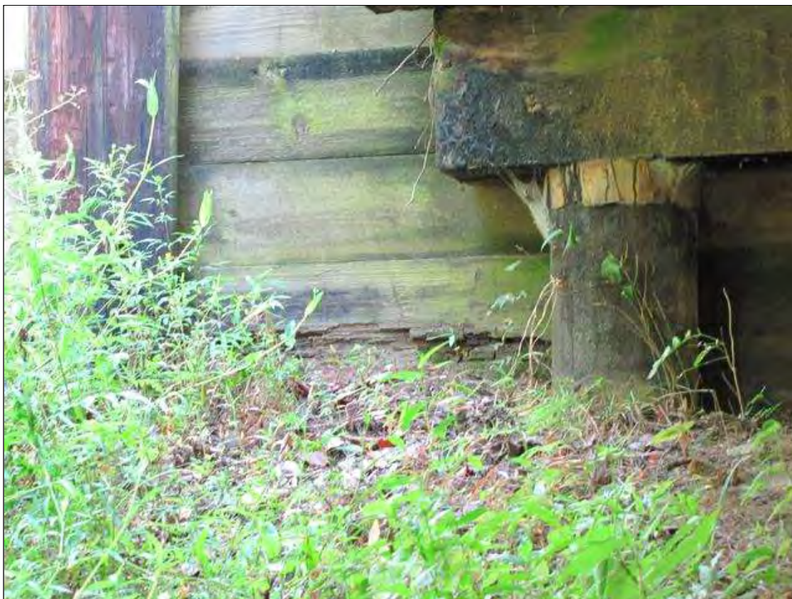
End Bent 2 Abutment/Backwall : 6 FT X 2 FT AREA OF DECAY AT LEFT SIDE AT PILE 1.
