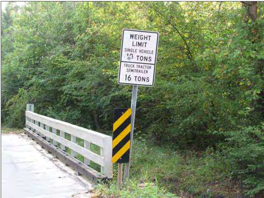
POSTING SIGN AT SOUTHEAST CORNER
