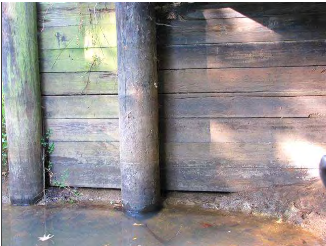
End Bent 1 Abutment/Backwall : 8 FT OF UNDERMINING AT RIGHT SIDE.
