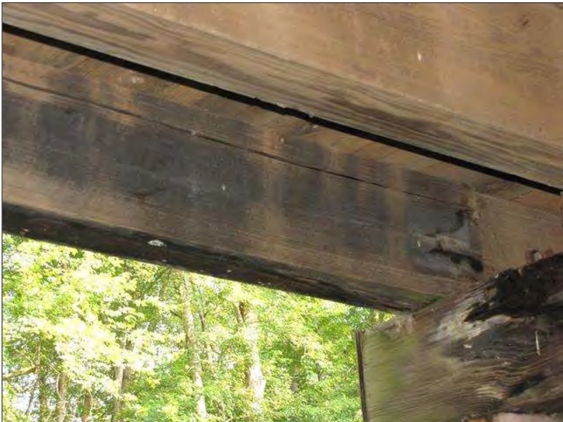
Span 1 Beam 1: SPLIT IN EAST FACE 3 IN FROM TOP, BEGINNING AT MIDSPAN TO BENT 1.
