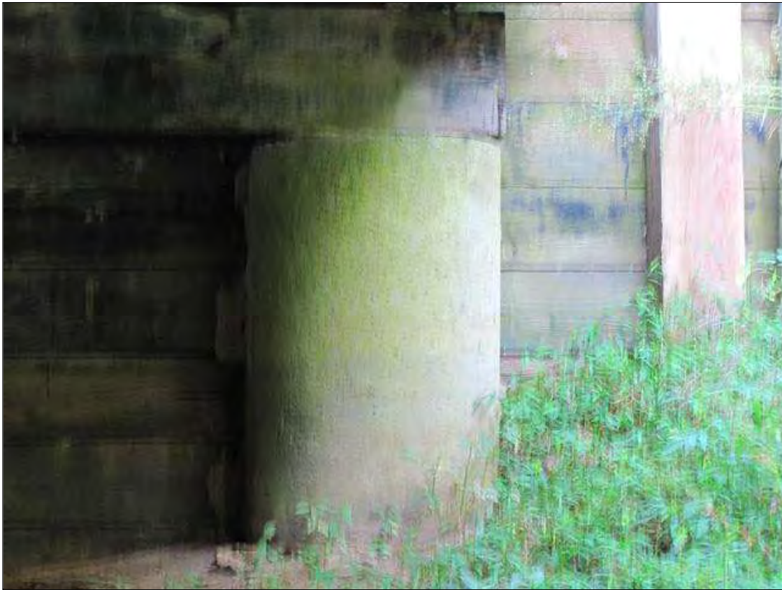
CONCRETE COLLAR AT PILE 1 END BENT 1.
