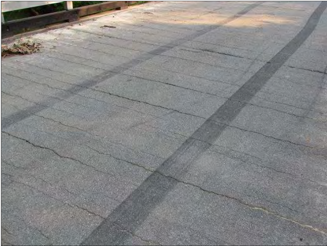
Span 1 Wearing Surface: TRANSVERSE REFLECTIVE CRACKS UP TO 1/4" WIDE THROUGHOUT WEARING SURFACE.
