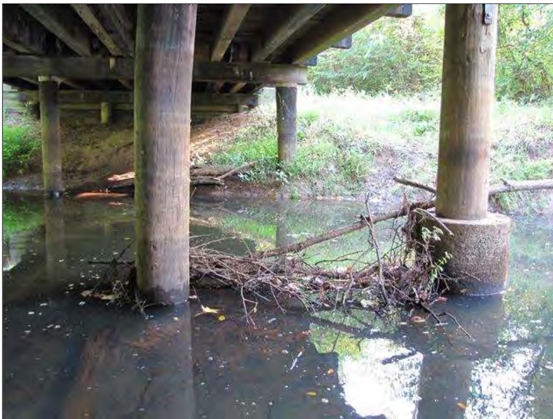
DRIFT ACCUMULATION AT BENT 1 BETWEEN PILES 3 AND 4
