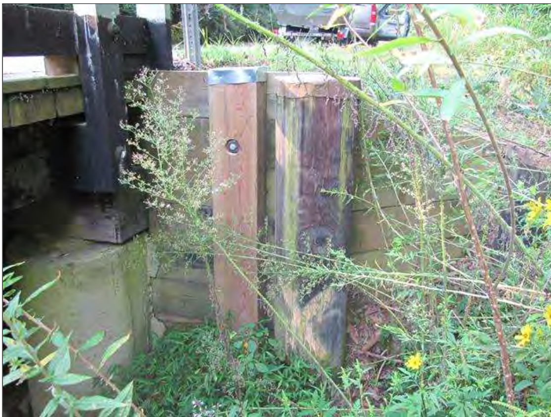
BULKHEAD REPAIR, WING PILE ADDITION AT LEFT SIDE OF END BENT 1.
