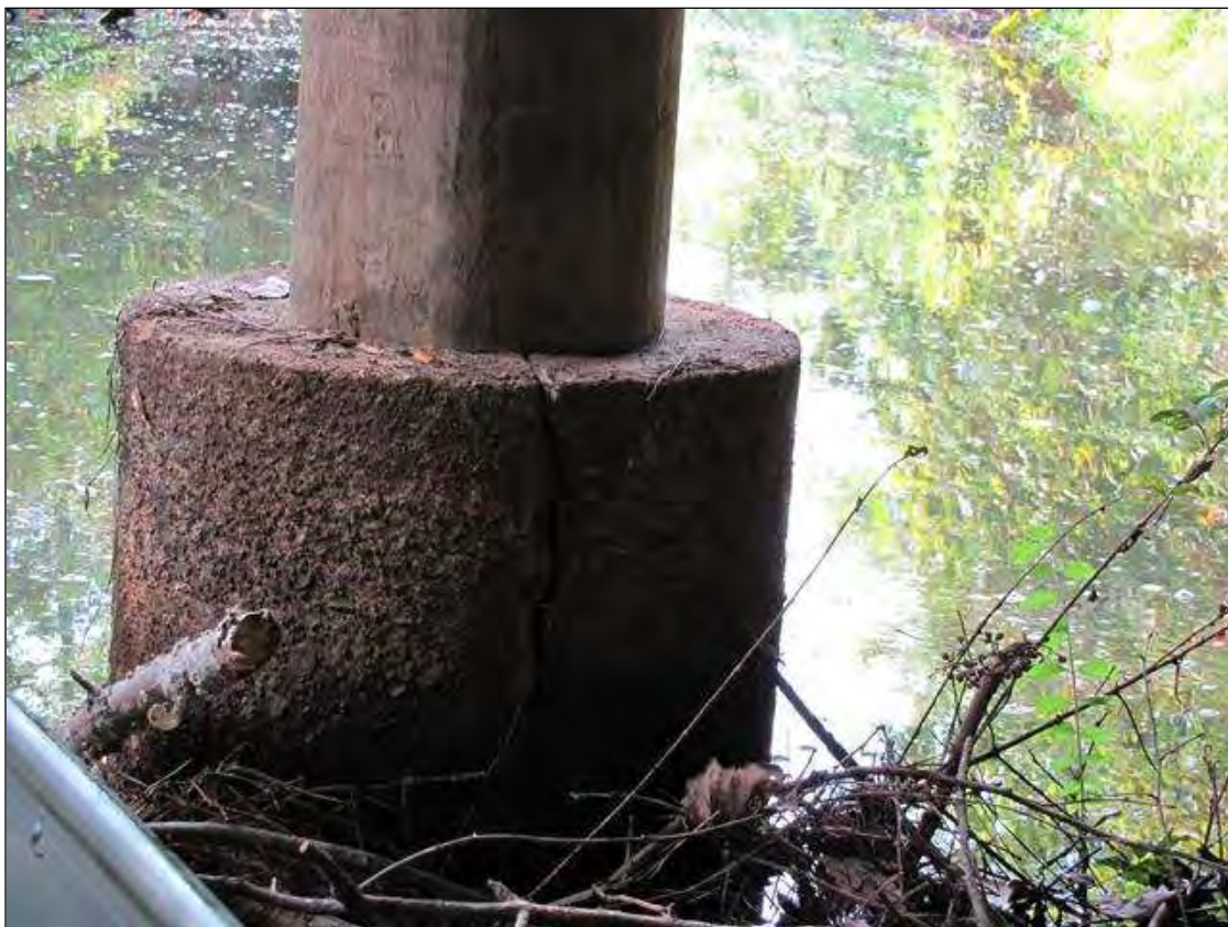
Bent 1 Pile 4: CONCRETE COLLAR IS CRACKED ON WEST FACE.
