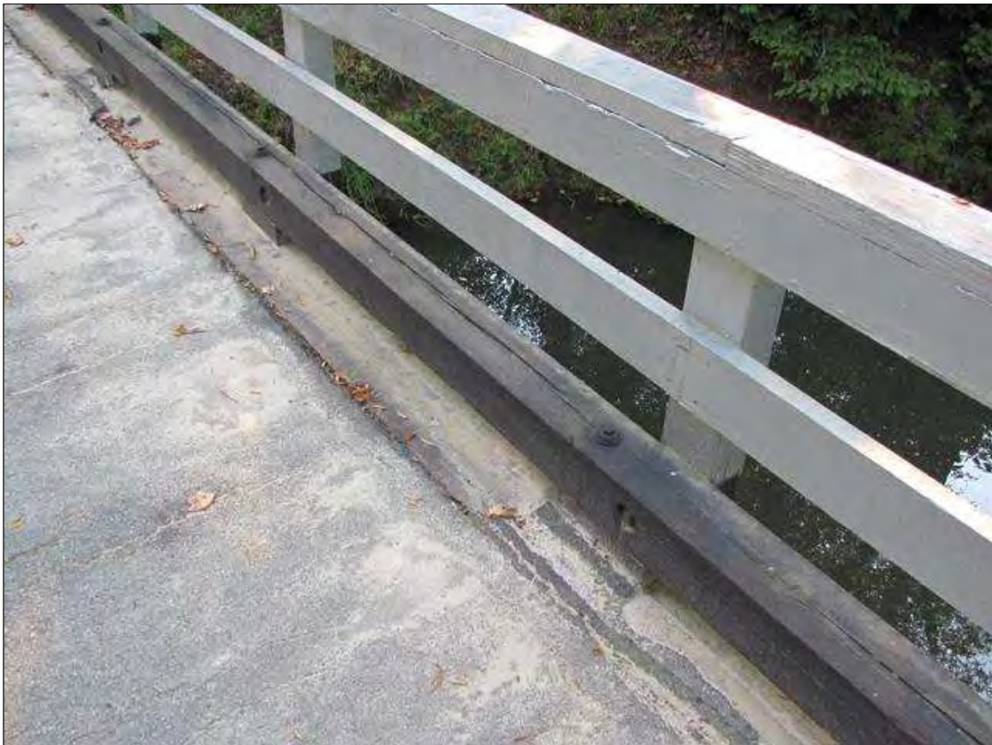
Span 1 Right Bridge Rail: FULL LENGTH CHECK IN TIMBER CURB.
