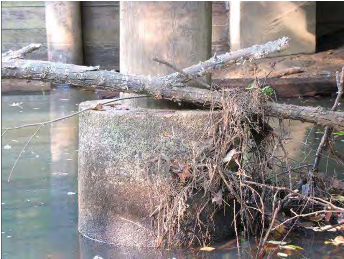
CONCRETE COLLAR AT PILE 4 BENT 1
