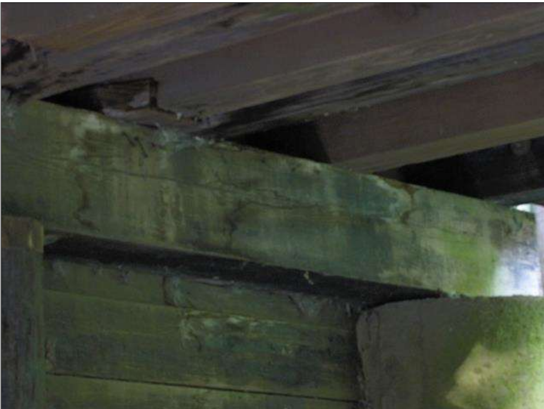
End Bent 1 Cap : RANDOM HORIZONTAL CHECKS THROUGHOUT CAP.
