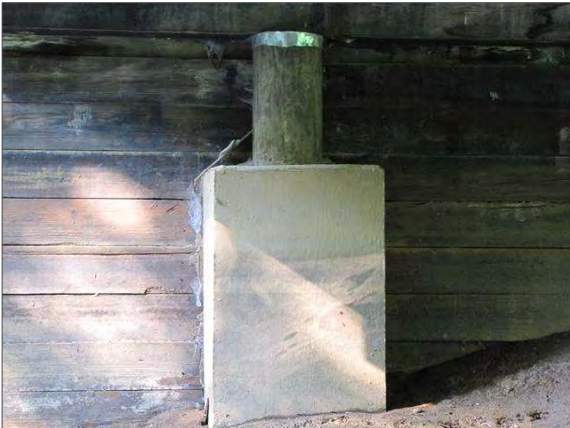
CONCRETE COLLAR AT PILE 3 END BENT 1.
